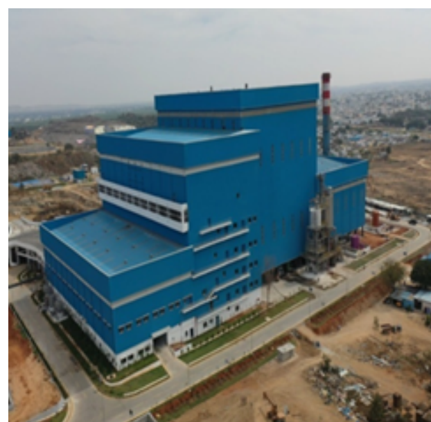
Waste to energy Plant at Jawaharnagar
